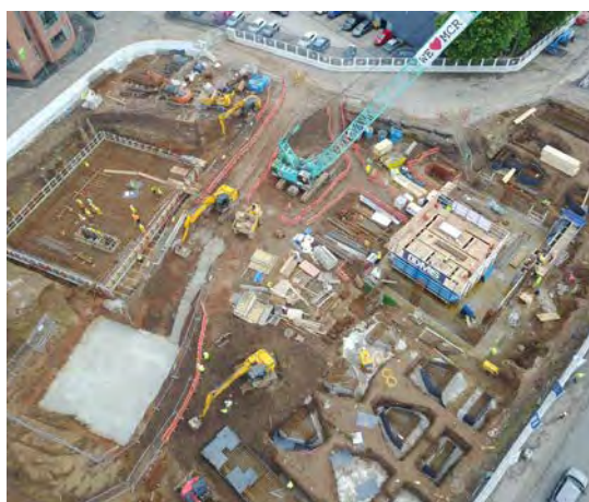
Figure 3.7: Drone picture of the Trinity Blackfriars project
